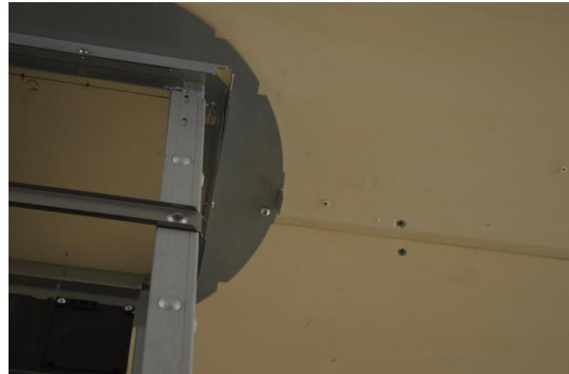
Install the hood on the ceiling by fixing, in addition to the 4 screws of the trestle, also the 2 of the upper tube support / installare la cappa al soffitto fissando con alter 4 viti al traliccio, alter 2 al tubo supporto tubo superiore
